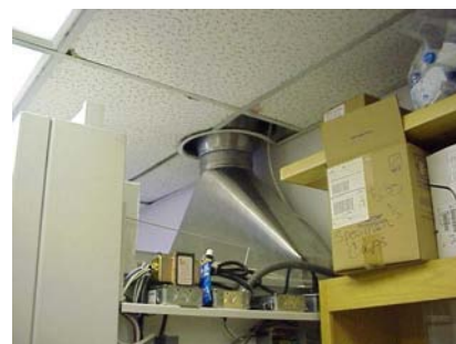
Figure 11. Exhaust duct connection.
