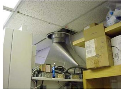
**Figure 11. Exhaust duct connection.**
