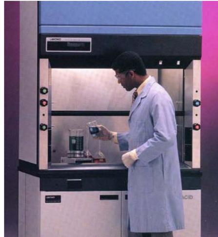
**Figure 1. Standard laboratory hood in use.**
